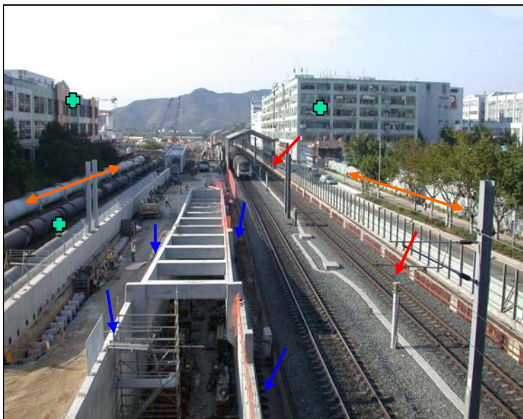
Typical on-site Geotechnical Instrumentation Locations
