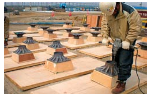
Fixing of casting at recess former
